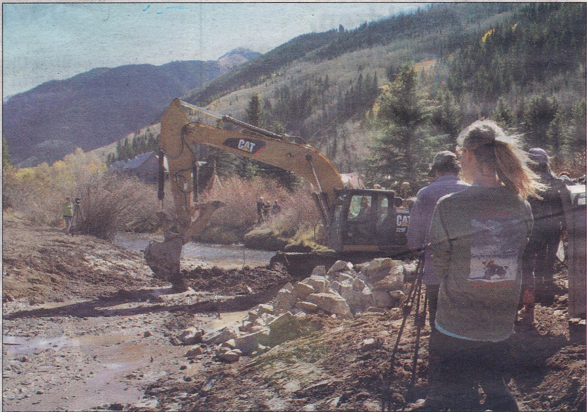
Onlookers watch as a bulldozer removes a dirt barrier allowing the San Miguel River to return to its original path as part of the Valley Floor River Restoration Project on Sunday. (Photo by Jessica Kutz)
