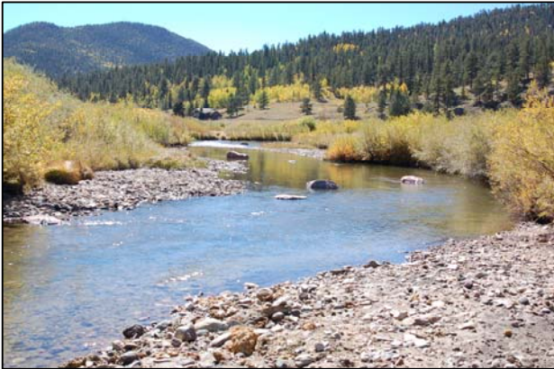
Photo 3 shows an example of a constructed bend-pool feature on Tarryall Creek in Park County. A constructed shallow riffle is evident in the foreground with a developed point bar (left) and bend pool (right). A slow water glide section is seen in the background. ERC project 2006.
